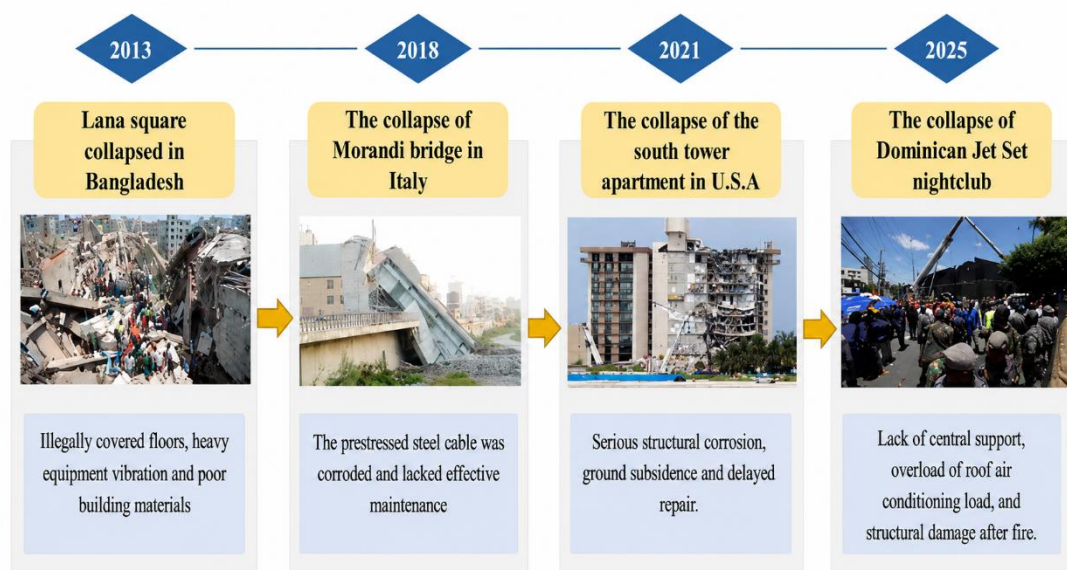
Figure 1. Accidents due to lack of structural health monitoring.
